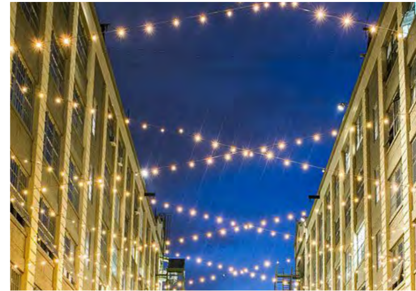
Bespoke catenary lighting to Fish Street
